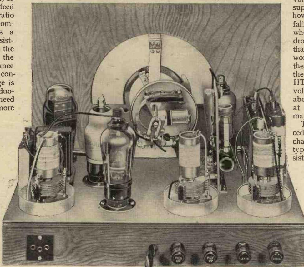
A rear view of the set with the coil screens removed.
