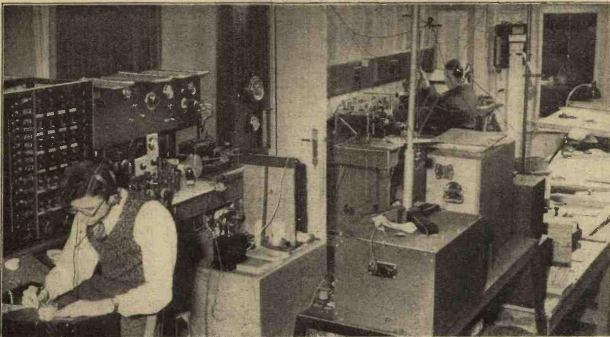
This general view of the interior of the checking station explains more eloquently than words the urgent need for more space. In the left foreground is the frequency measuring gear; behind the engineer is the apparatus for measuring modulation. In the background is the field strength "explorer."
