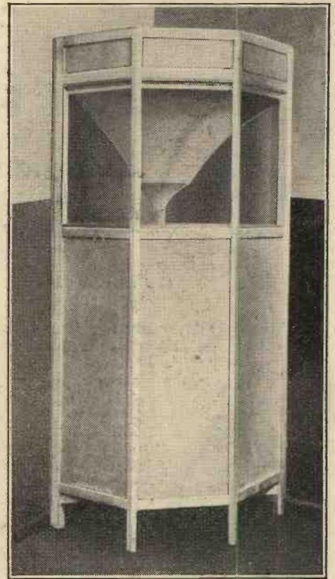
Designed to fit into a corner of the room, the latest Voigt domestic loud speaker retains the acoustic characteristics of its large-sized "straight" horn equivalent.
