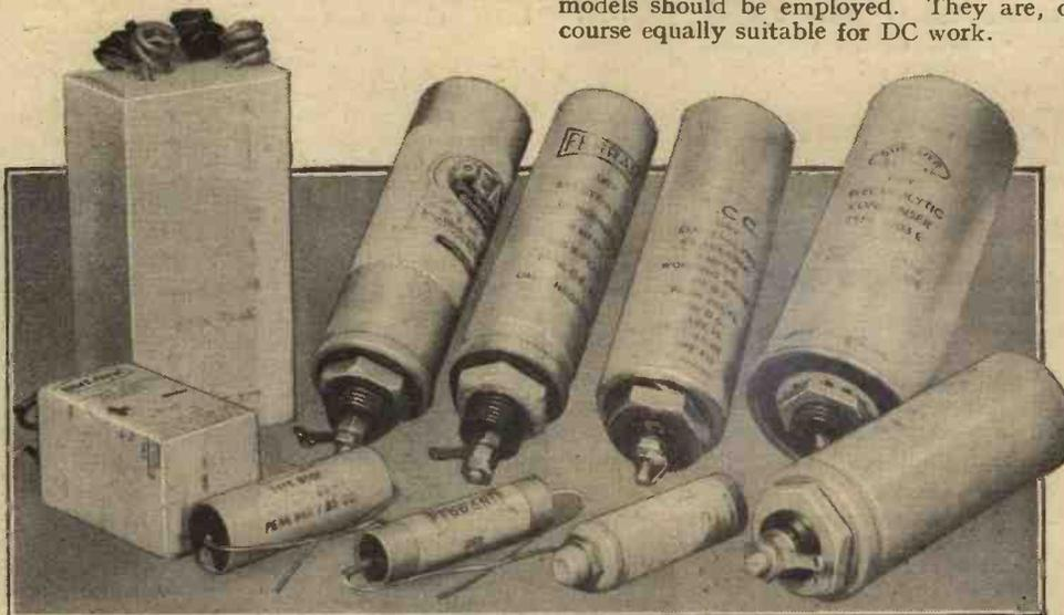
(C) Typical modern electrolytic condensers comprising Ferranti; Bulgin; Peak; T.C.C.; Dubilier and Polar-N.S.F. models. The small tubular types are for grid bias de-coupling circuits.
