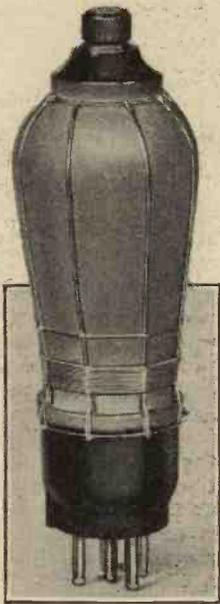
A loose valve base secured by a wire binding.
