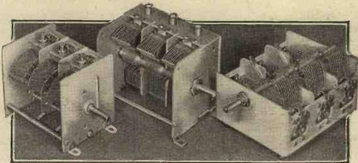
A group of three-gang condensers; the ones on the left and right are, respectively, Polar and J.B. straight condensers, while that in the centre is a Utility superheterodyne model.
