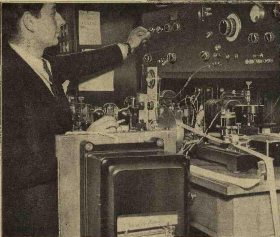
M. Boulanger, head of the checking department, with the apparatus used for measuring and recording the modulation depth of every European broadcasting station.
