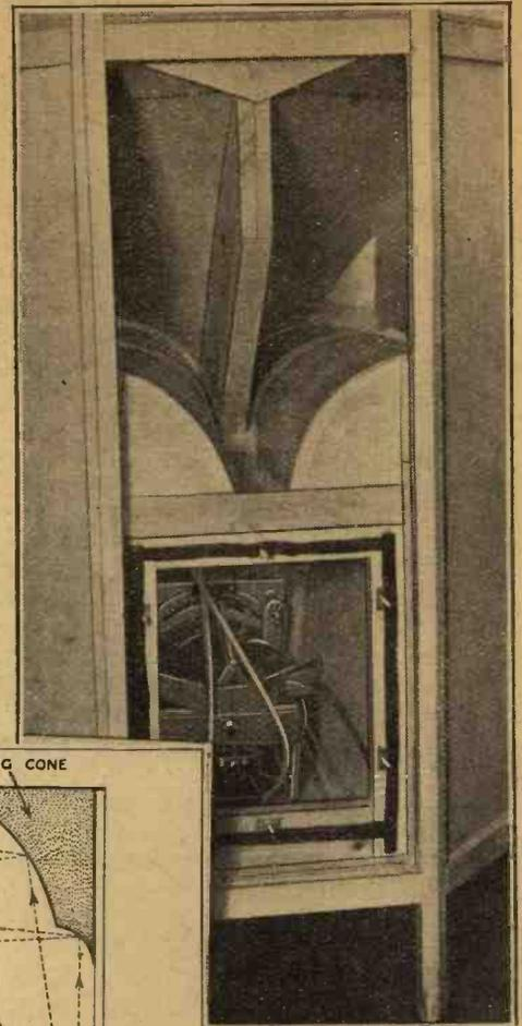
Front panels removed giving access to the bass-chamber and twin-diaphragm unit, and (left) diagrammatic section of cabinet, showing alternative sound paths.
