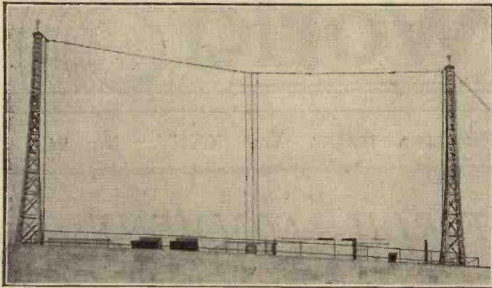
Two aerials used for ultra-short-wave broadcasting in the London district. Above is the five-metre aerial on Broadcasting House. (Right) The di-pole aerial used by the Baird Company in television experiments at the Crystal Palace.
