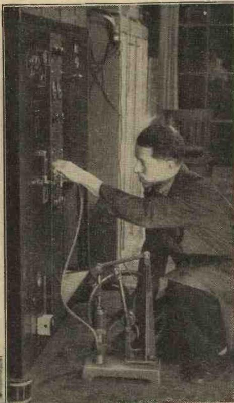
An engineer checks the pressure in the chamber containing the tuning fork which provides the frequency standard for calibrating wavemeters.
