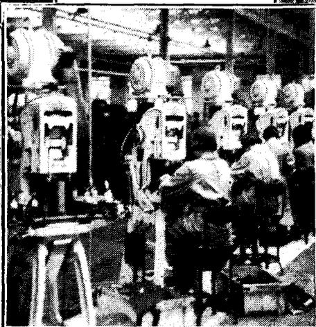
Here nuts, screws and spindles are turned out by the automatic lathes, while coil cans, laminations, switch contacts, etc., are produced by the automatic toggle presses. A huge automatic cadmium-plating plant has just been installed in which a chain conveyor takes the chassis parts through cleaning and washing baths, and, after passing at a regulated speed through the plating vat, finally dries the products in a hot-air oven at the far end.
