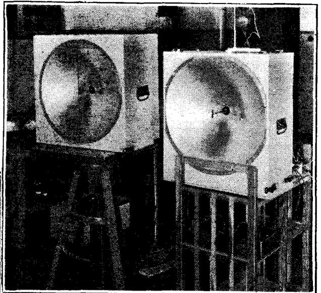
Ten-centimetre beam transmitter and receiver with reflectors.
