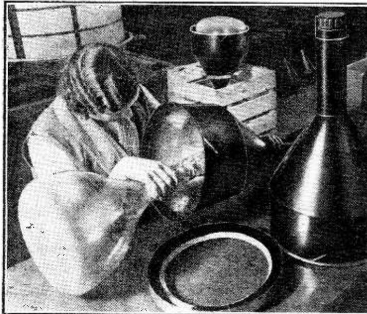
Cathode-ray tubes for television receivers being fitted inside metal screens at the Osram-G.E.C. lamp works.
