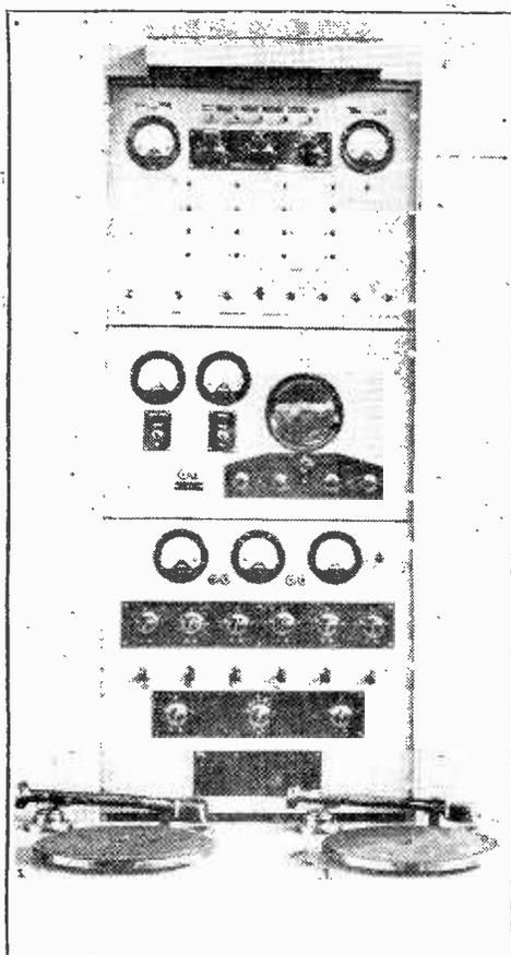
Marconiphone PA equipment fitted with dual turntables.
