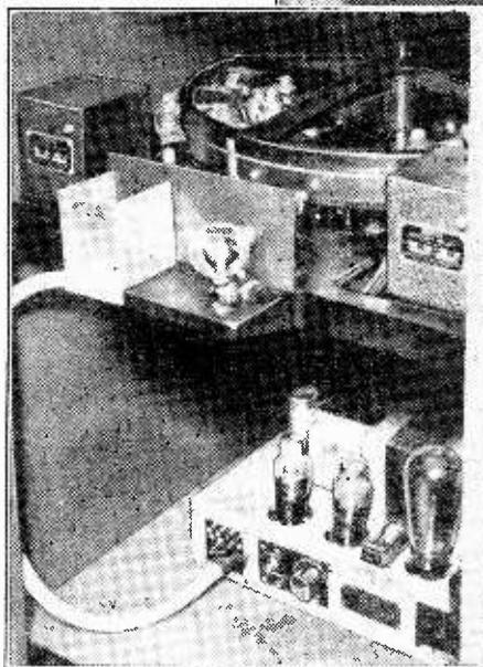
Station. By means of loud speakers passengers are warned to "Stand Clear of the Doors" before these are automatically operated. The system employs an amplifier and a photo cell fed from a controlled sound track on a continuous belt of film, illuminated by a 12-volt lamp. A spare lamp automatically comes into operation should the original one burn out.
