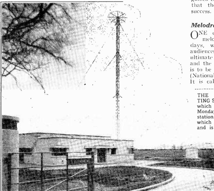
THE PENMON TRANSMITTING STATION near Beaumaris which was officially opened on Monday last. A feature of the station is the 250 foot mast which itself acts as the aerial and is surmounted by a capacity ring 40 feet in diameter. The power of the transmitter is 5 kW. The transmissions are on the same wavelength (373.1 metres 804 kc/s) as the West Regional at Washford to which station the frequency is synchronised.
