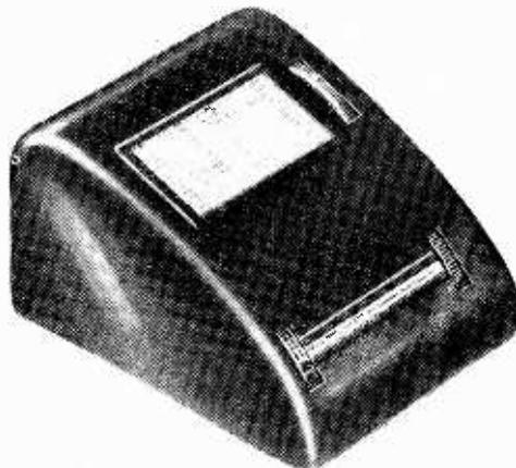
STATION-FINDING MADE EASY.—This "rotary station log" contains a 12-ft. length of tape, on which is printed information relating to over 1,600 broadcasting stations throughout the world. Stations are listed in order of frequency, and, as the device is of American origin, in order of call-signs as well. One knurled disc rotates the drum carrying the tape, while the other controls an indicator showing standard zone time.
