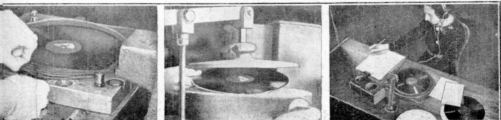
of the press, the faces of which automatically come together with a pressure of 64 tons. Steam circulates between the matrices, followed by a rate or so, after which specially trained girls test the first record off each pair of matrices before further copies are made.
