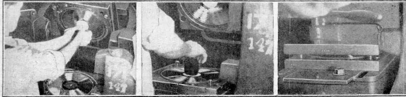
Next we see the appropriate record labels being placed on the upper and lower matrices in the press, and the rolled "biscuit" is placed in the press and cold water for cooling, and the record is ready to be withdrawn. The record is then placed under the cooling press for a
