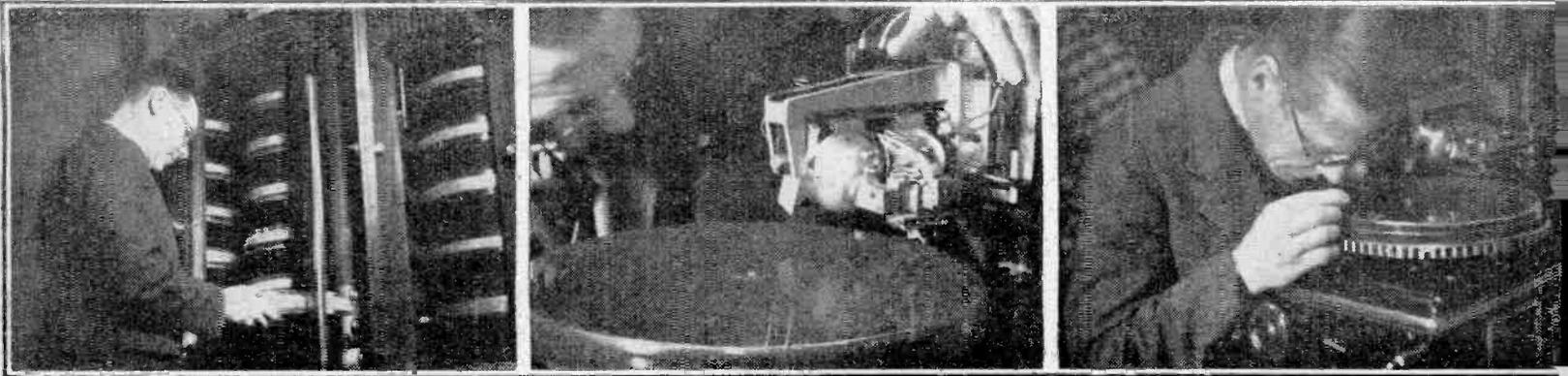
Wax blanks are kept in a specially heated store, from which one is removed when everything is ready for a record to be made. A few test grooves are cut; the weight used to rotate a turntable carrying the wax; the weight used for this machine is shown in the fourth picture above. Whilst the record is being cut, the recording instrument is lifted from the wax and the
