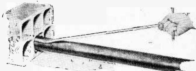
A socket wrench with a universal joint to reach normally inaccessible points has been produced by the Bell Telephone Laboratories of New York City.
