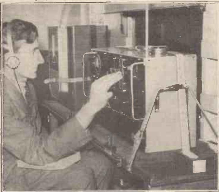
**RADIO NORMANDIE'S FIELD STRENGTH.** One of the engineers adjusts the Marconi-Ekco field-strength measuring set in the International Broadcasting Company's Reception Test van which is surveying the service area of the new 20-kW Radio Normandie Station at Louvetot.
