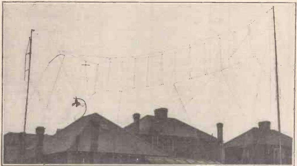
The imposing array of aerials at G6OT. A multi-element directional system for five-metre transmission can be seen suspended between the two masts.
