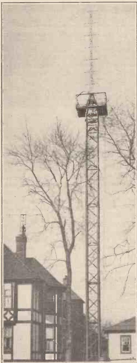
The "turnstile" aerial at W2XCR, formerly W2AG, at Yonkers, N.Y. It comprises 14 sections and is supported by a 100ft. tower.
