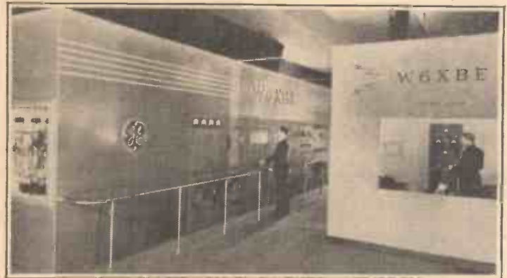
TREASURE ISLAND'S 20-kW short-wave transmitter, W6XBE. Erected in the Palace of Electricity at the San Francisco Golden Gate International Exposition, it radiates transmissions to the Far East on 9.53 Mc/s., when the path between the transmitter and the destined listening point is dark and on 19.57 Mc/s. when part of the path is light.
