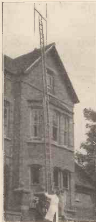
Erecting the demonstration aerial.
