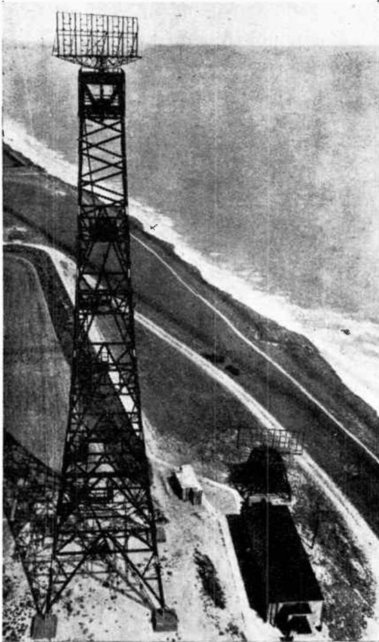
Rotating beam arrays used at CHL stations. The 185-ft. tower is used at sea level and the 20-ft. gantry shown on the right is for installation on cliffs.
