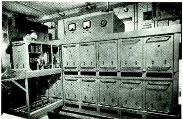
A section of the Wayne Kerr multiple-unit transmitter is shown withdrawn from its housing on the trolley provided for maintenance.
