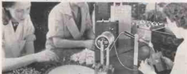
Soldering capacitors at A. H. Hunt Limited. The capacitors are heated together with short pre-cut lengths of *Ersin Multicore*.
