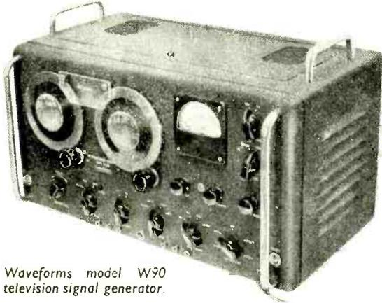
Waveforms model W90 television signal generator.
