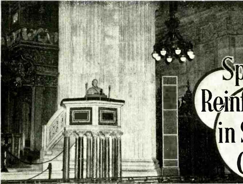
Vertical loudspeaker column for the dome area mounted to the right of the pulpit.
