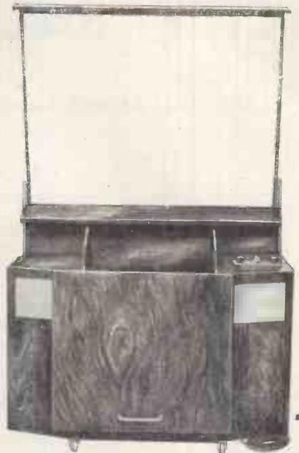
The above photograph shows the receiver closed, in this position it may be securely locked. On the right the receiver is shown opened for viewing. Note the remote control panel on the right hand side of cabinet.
