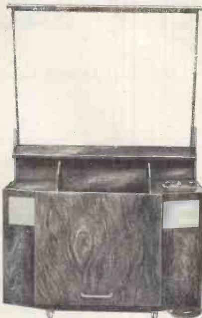
The above photograph shows the receiver closed, in this position it may be securely locked. On the right the receiver is shown opened for viewing. Note the remote control panel on the right hand side of cabinet.
