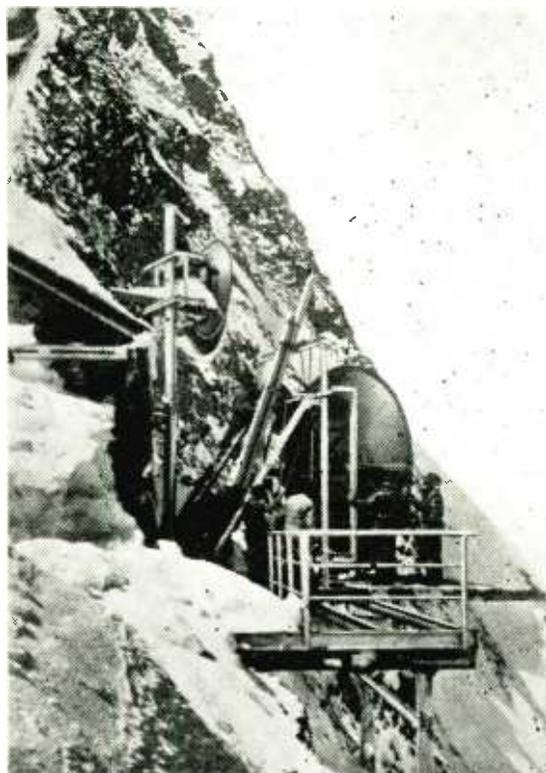
Paraboloids, each weighing half-a-ton, being erected at the Jungfrau relay station. (See "Trans-European TV")
