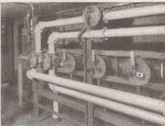
Coaxial feeder switching equipment in an upper room of the station. The functions of the coaxial switches here can be seen in Fig 1.
