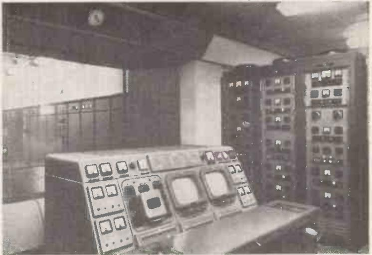
Main control desk, with a view through the window of the transmitter hall. The cubicles on the right contain the crystal-drive and phasing equipment.
