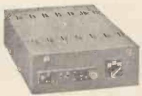
Type BM2. Size 8 x 5 1/2 x 2 1/2 in. Supplies 120 v., 90 v., and 60 v., 40 mA, and 2 v. 0.4 a. to 1 amp. fully smoothed. THEREBY COMPLETELY REPLACING BOTH H.T. BATTERIES AND L.T. 2v. ACCUMULATORS when connected to A.C. mains supply 200-250 v. 50 c/s. SUITABLE FOR ALL BATTERY RECEIVERS normally using 2 v. accumulator. Complete kit with diagrams and instructions 49/9 or ready for use 59/6.
