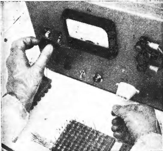
**TRANSISTOR MANUFACTURE.**—This photograph, taken at the new Mullard Southampton works devoted entirely to semi-conductors, shows preliminary testing of a transistor before final enclosure. To prevent contamination, the test is made in a sealed "dry box."
