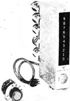
allows the selection of a digit between 0 and 9, but several of the devices can be connected in cascade to count units, tens, hundreds, thousands, etc., and the same method of pre-selection is applied to them all. A rotary switch at the end of a five-wire cable is used for the remote pre-setting of each decade.
