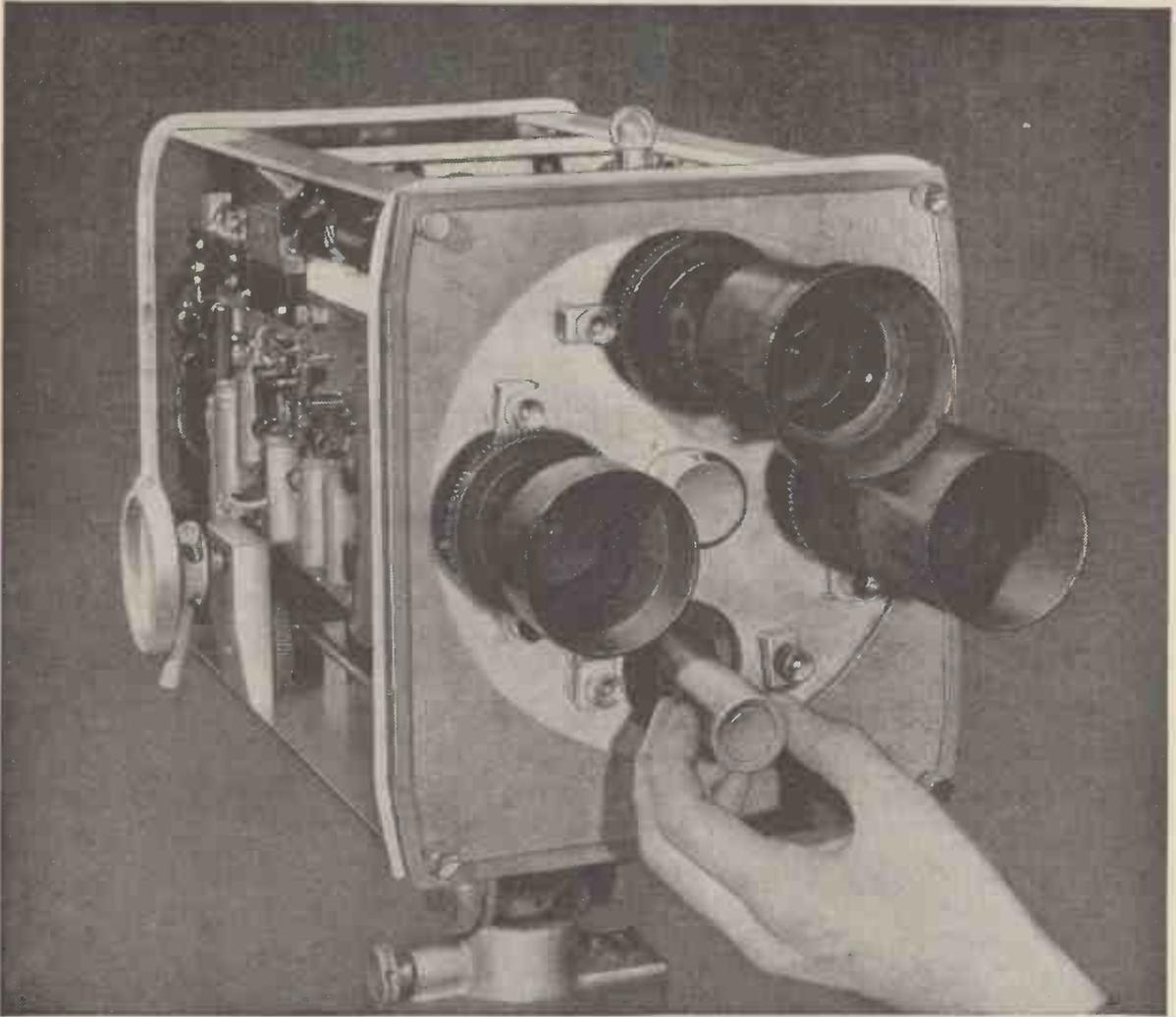
Camera Type 201 with panels removed illustrating accessibility
