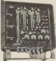
Offered at about one-twentieth of original cost. This is an ex-Government switchboard. It contains three reverse current relays, one voltmeter, one main ammeter, two secondary ammeters and three variable resistors for controlling circuits. These are original cases. Price 22/15/-. Carr. 10/-.
