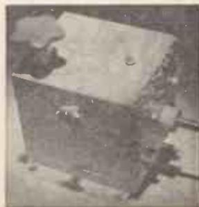
instantaneous reverse at any speed. Recommended input speed 500-1,000 r.p.m. maximum power 1 $\frac{1}{2}$ h.p. Both shafts  $\frac{1}{2}$ in. dia. with Woodruff key.
