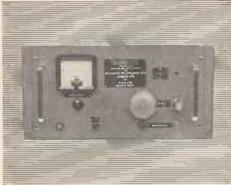
This E.H.T. Cable Insulation Tester has been designed and made for detecting and recording faults in the insulating coverings of cables during manufacture. The system permits a very high speed of operation.
