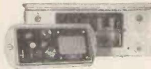
Type 70 (replaces Type 715) 15 watt V.H.F. mobile Transmitter/receiver for boot mounting. The control unit may be removed and used as Extended Control mounted on the dashboard. On the multichannel version up to six adjacent channels are available and may be remotely switched.
