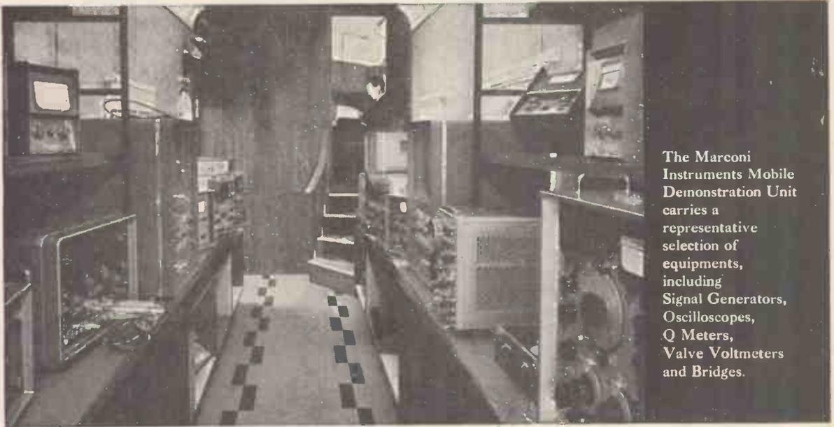
The Marconi Instruments Mobile Demonstration Unit carries a representative selection of equipments, including Signal Generators, Oscilloscopes, Q Meters, Valve Voltmeters and Bridges.
