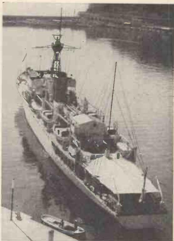
Fig. 4. British Naval Survey Ship equipped with Two-range Decca showing tubular aerial mast for transmission of the master signal.
