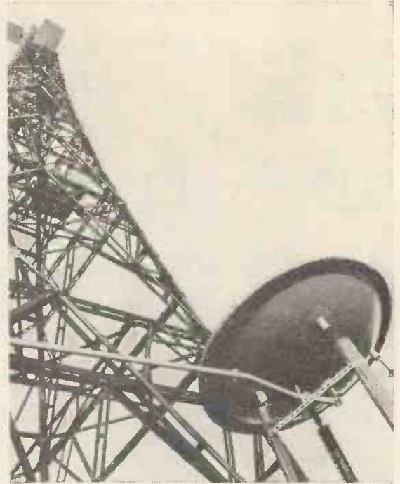
Plane passive reflector on mast reflects to next repeater beam from aerial at ground level.
