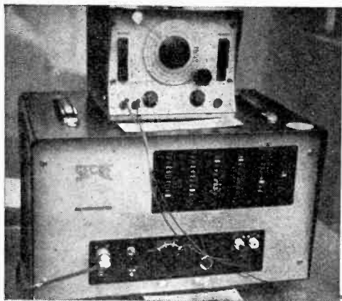
Transistor a.f. generator and transistor frequency meter (0 to 1 Mc/s) shown by S.E.C.R.E.
