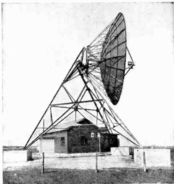
Experimental tropospheric scatter station at Start Point: frequency 858Mc/s, power 10kW.
