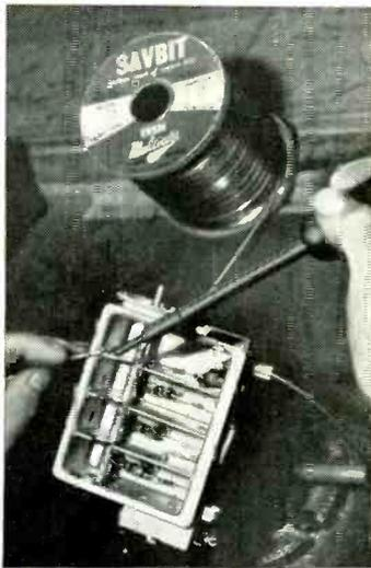
**H. J. Leak & Co. Ltd.** Ersin Multicore Savbit alloy is shown in use in the wiring construction of the Leak Integrated Stereo 30 Transistor Amplifier. In order to ensure the utmost reliability, the Leak High Fidelity equipment has been made with Ersin Multicore Solder for more than 20 years.
