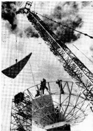
*The aerial structure for the satellite earth station on Ascension Island in the South Atlantic to be owned and operated by Cable and Wireless Ltd. has been set up for tests on the Marconi radar test site at Rivenhall, near Witham, Essex. The aerial structure is undergoing nearly two months of overall testing before being shipped to Ascension, and COMSAT has agreed to loop tests being conducted with the Early Bird satellite.*
