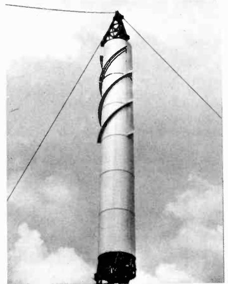
*The upper section of the television aerial system for the new mast at Emley Moor undergoing tests at E.M.I. The aerial system, which is 180ft long, will be hoisted up the centre of the 900ft concrete mast. The helical strakes are designed to reduce mechanical oscillation under severe wind conditions.*
