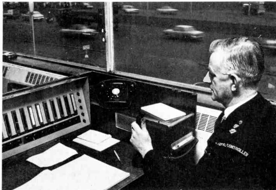
*The traffic control room at the Dartford tunnel. S.T.C. have recently installed a single-channel u.h.f. communication system which allows contact with service control vehicles. The use of u.h.f. has overcome the problems of receiving the signal inside the tunnel itself and no dead spots exist at the tunnel mouths due to cancellation effects.*
