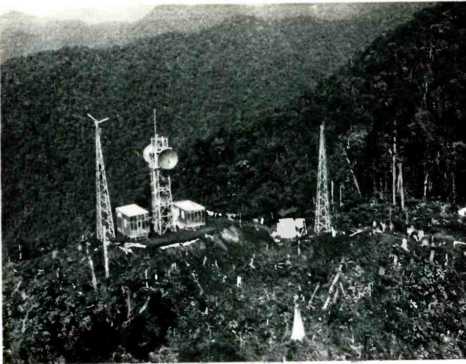
*Receiving and transmitting aerials of telecommunications equipment designed by Page Communications Engineers which links the copper mining operations on the island of Bougainville with the mainland of New Guinea.*
