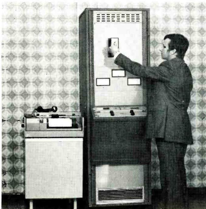
Complete prototype colour telephoto transmitter.
