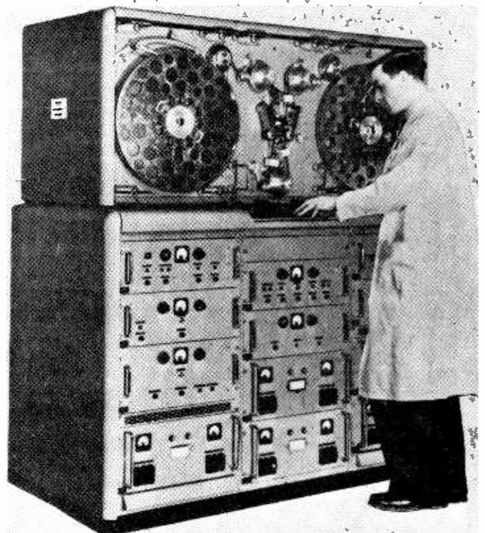
ic tape record was first demonstrated to members of the Press.<sup>55</sup> This was a two track stereo recording initially mastered at 15 i.p.s. and then duplicated down to 7.5 i.p.s. for domestic consumption.
