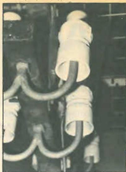
Fig. 9. Simple and effective conical skirts of common British telegraph pole insulators, in use for nearly a century, and only now recently adopted for marine use, Figs. 10 and 11.
