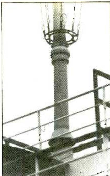
**Fig. 11.** Base of Russian mast showing three deep-skirted rain cones on the central glass-fibre pole. (Photographed at Rcuen, 1983.)
