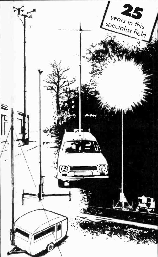
The smoothly operated QTM Mast comes fitted with handpump or can be vehicle mounted with 'Power Pack' for extension and retraction. Available in a range of heights up to 15 metres, the QTM mast can provide the ideal answer for:
