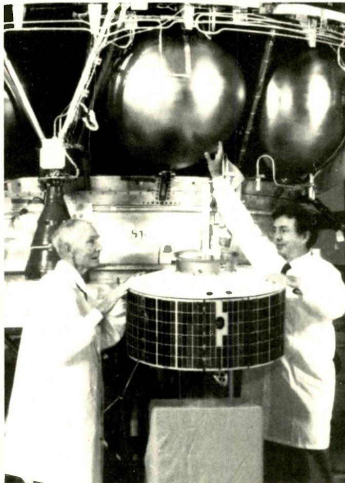
Pioneer Dr Harold Rosen (left) with the prototype of his Syncom, the first geostationary communications satellite. A colleague, Tom Hudspeth, points to one of the fuel tanks of the new Intelsat VI which stands behind in the Hughes plant at El Segundo, California. Syncom, weighing only 35kg, would fit inside this tank. Intelsat VI is 120 times heavier at 4240kg.
