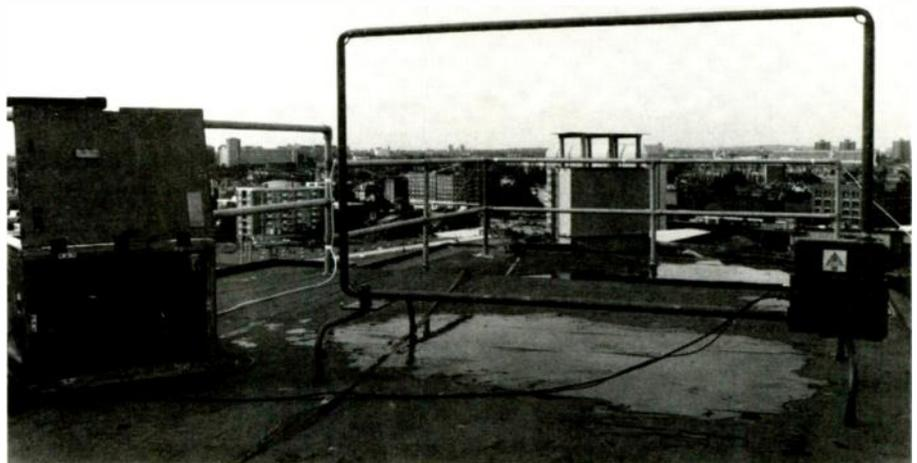
**Minimal size HF transmitting aerial developed by British Aerospace. This collapsible loop of extruded aluminium will handle 400W and comes complete with automatic tuning unit.**
