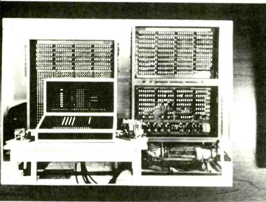
*The reconstructed Z3 computer at the Deutsches Museum, Munich. Left, memory unit; right, control and arithmetic unit; front, keyboard/display with paper tape reader to the right. In the original were two cabinets for the memory unit, each measuring about 6×3×1 feet.<sup>2</sup>*
