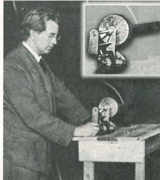
Fig. 4. John Logie Baird in 1927 at the Leeds demonstration to the BA. He is posing with a wax cylinder video record/playback system – the precursor to 'Phonovision'. The drive shaft probably connected the Nipkow camera disc with the cylinder drive. No cylinder recordings have survived.
