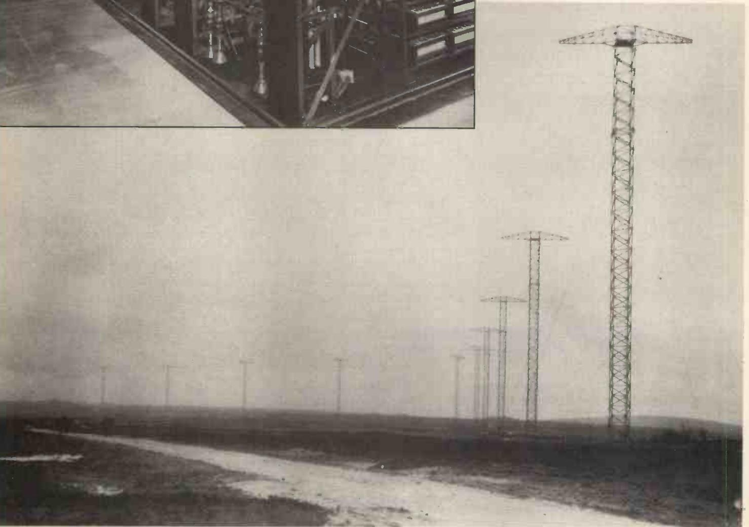
The shortwave Imperial wireless chain – the beam system as it came to be called – like its long-wave high power predecessor was based on pairs of stations, a transmitter and receiver. Many were in fact conversions of stations begun for high-power links.
