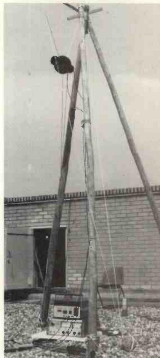
*Transmit site antenna support at the University of Surrey, with CFA horizontally polarised. The support stands approx 4m high on the flat roof of a five storey building.*
