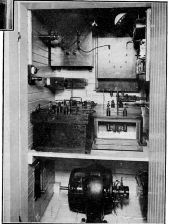
*The Transmitting Apparatus in a Silence Cabin.*
