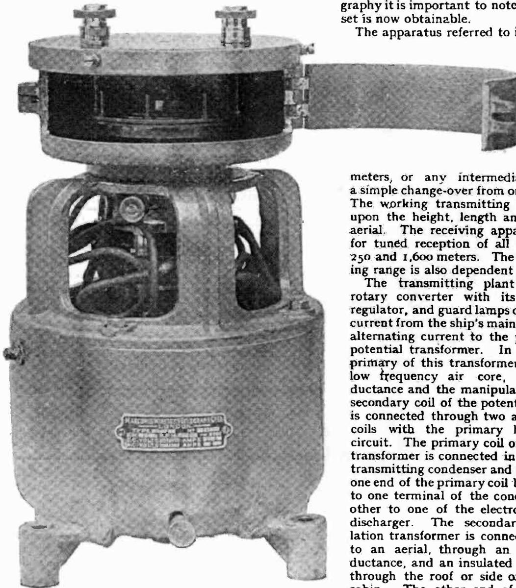
$\frac{1}{4}$  k.w. Converter with Disc Discharger.
