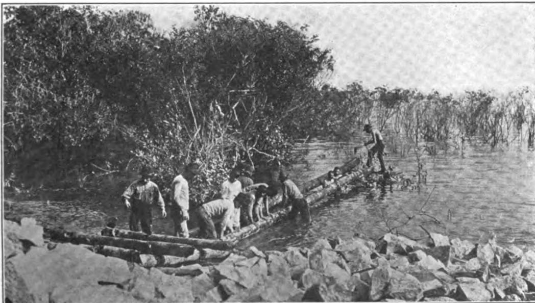
*The Bank Commenced to Slide Rapidly and Before All the Material Could Be Unloaded the Track Had to Be Extended on Trestles.*
