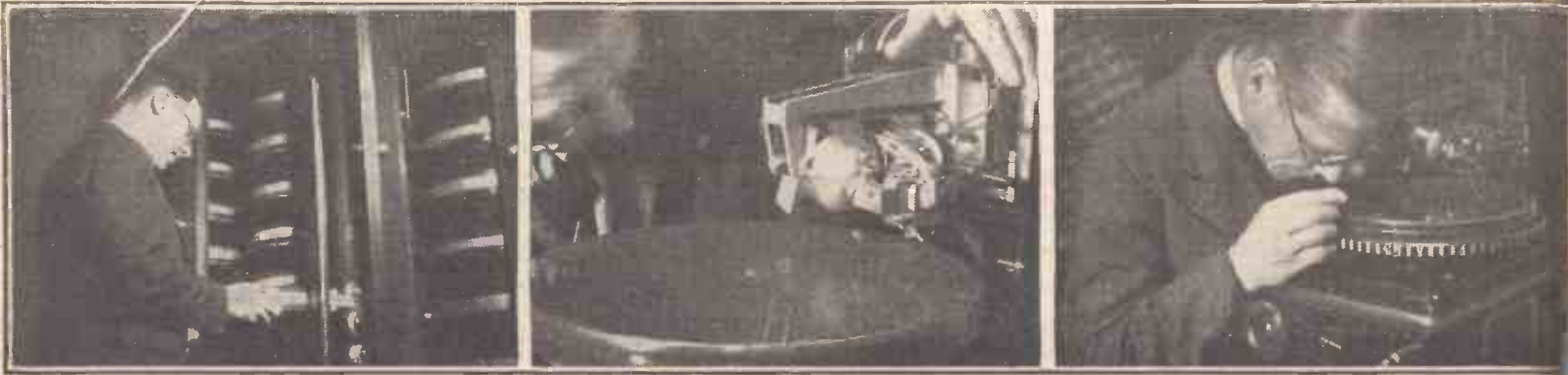
Wax blanks are kept in a specially heated store, from which one is removed when everything is ready for a record to be made. A few test grooves are cut with is employed to rotate a turntable carrying the wax ; the weight used for this machine is shown in the fourth picture above. Whilst the record is being cut the recording instrument is lifted from the wax and the
