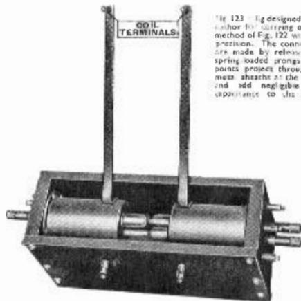
Fig. 123—Fig. designed by the author for carrying out the method of Fig. 122 with high precision. The connections are made by releasing the spring loaded prongs whose points project through the mesh sheath at the centre and add negligible stray capacitance to the circuit.
