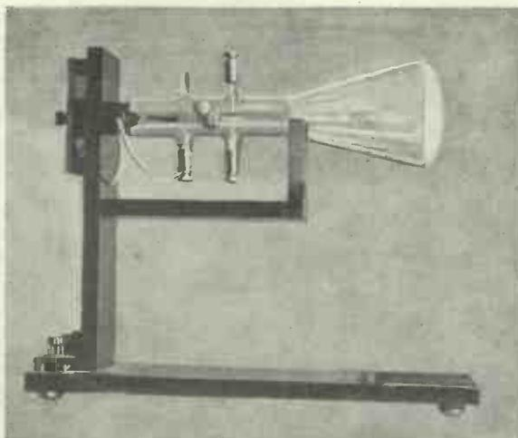
The "fluorescent" coating can be seen as a white surface on the end of this cathode-ray tube.
