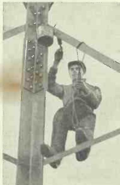
*Radio masts need an overhaul in the Spring just like the home. But painting the masts, four or five hundred feet above the ground, is a "he-man's" job, and if it's very windy—! The workman seen here is at work on the Warsaw station.*
