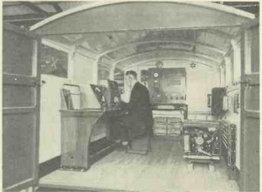
*The importance of radio to aircraft increases with the expansion of flying. When a new station is proposed, tests are carried out over several months with a portable station in a motor "trailer," such as the Marconi equipment illustrated above. These trailers have been in use at Hull, Belfast and Portsmouth.*
