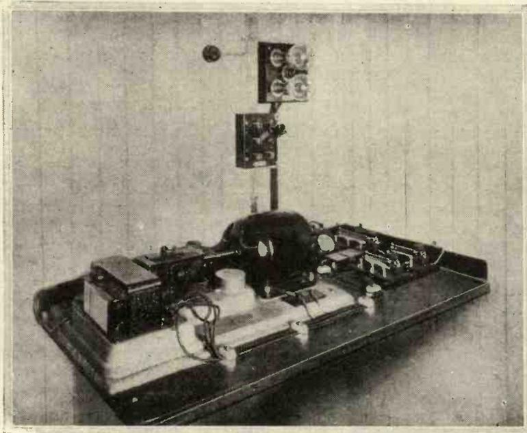
Fig. 3.—The Wheatstone high-speed automatic transmitter.
