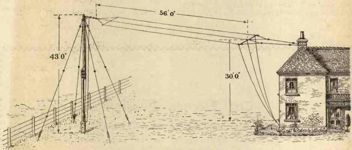
Fig. 1.—The aerial completed and ready for use.
