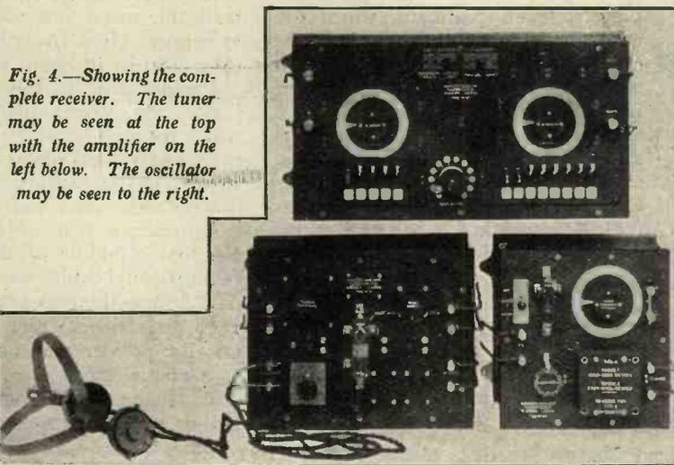
Fig. 4.—Showing the complete receiver. The tuner may be seen at the top with the amplifier on the left below. The oscillator may be seen to the right.
