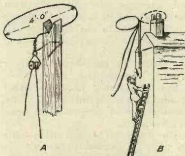
Fig. 19.—Method of lifting loop over chimney.
