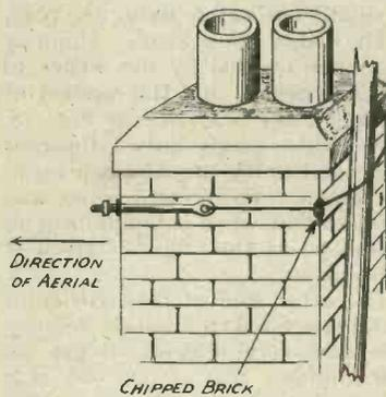
Fig. 16.—Method of fixing pole.
