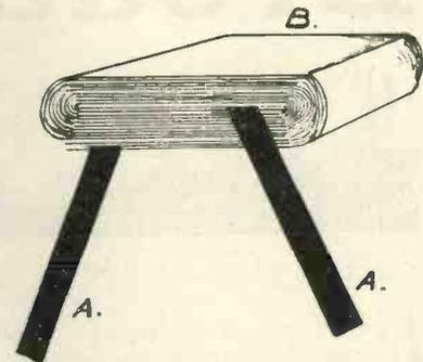
Fig. 11.—Condenser after pressing.
