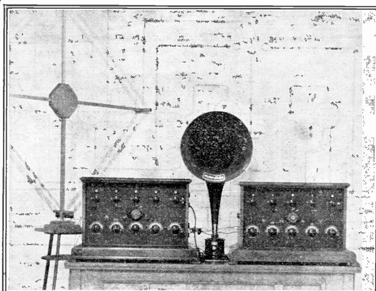
*Fig. 3.—The "Super 5," together with the super-heterodyne, makes a very interesting and efficient installation. Note the frame aerial.*
