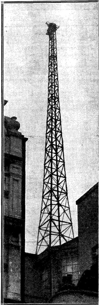
*On and after February 14, 2LO will transmit from a new and improved aerial on the roof of Selfridge's, in Oxford Street. The aerial hitherto used has been that belonging to the Marconi Company on Marconi House, but owing to its proximity to the Air Ministry's aerial on Adastral House, with which it has interfered, its further use for broadcasting is prohibited. Our photograph shows the new mast on Selfridge's roof.*
