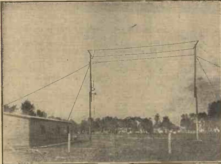
The masts and aerial at the Westinghouse Electric Manufacturing Company's station at Hastings, Nebraska. The call letters are KFKX.
