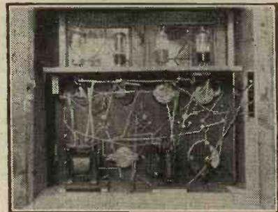
The wiring of Mr. Hubbard's receiver.
