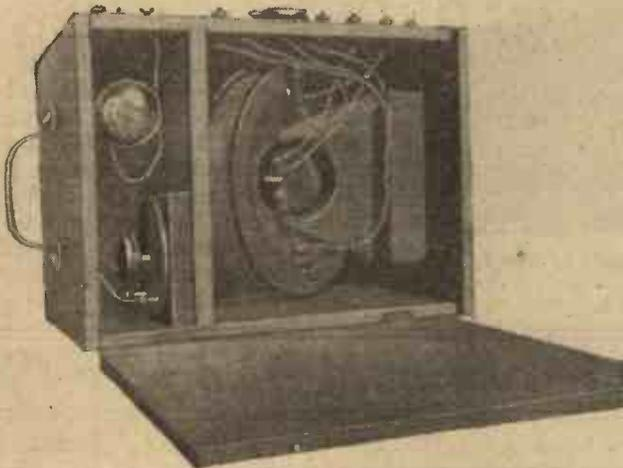
*The oscillator used in these experiments was designed for low frequencies. The valve may be seen in the compartment on the left.*
