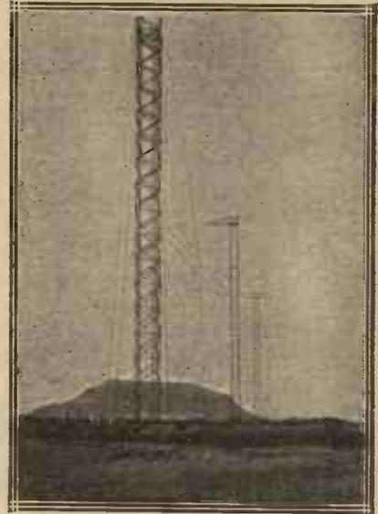
The great beam station near Poona, in India, is making rapid progress. The five masts are each to be 297 feet high, and they are being sent out from England in sections. They are 12 feet square and the cross arms are 20 feet long.
