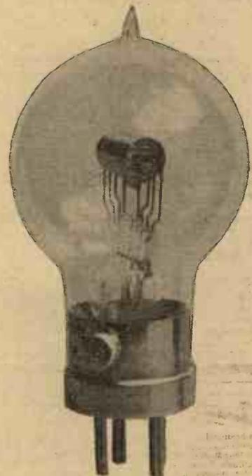
This double-grid valve, which is a product of Messrs. Radio Valves, Ltd., employs a terminal on the metal cap for connection to the inner grid.
